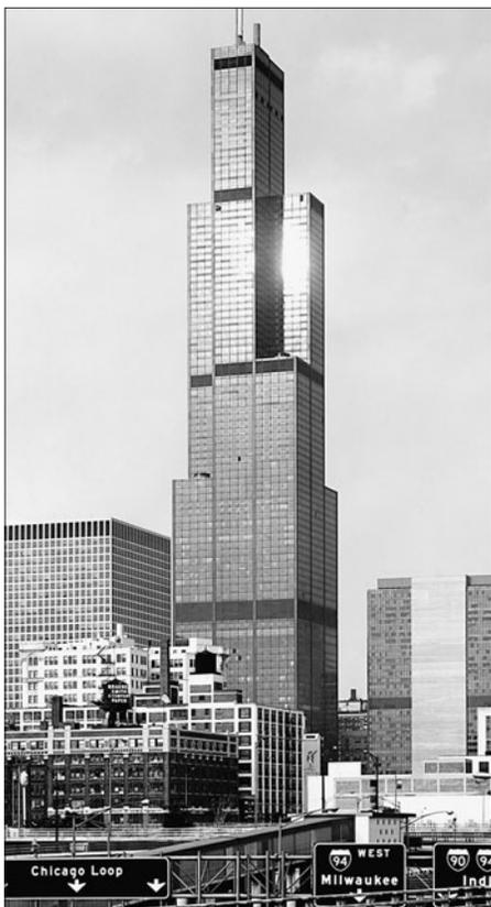
Fig. 2: 442 m Sears Tower introduced the bundled tube system (Ezra Stoller<sup>®</sup> Esto)
