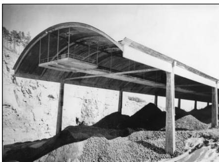
Fig. 3: Shell roof; 30 × 168 m, height – 18 m, Norway
