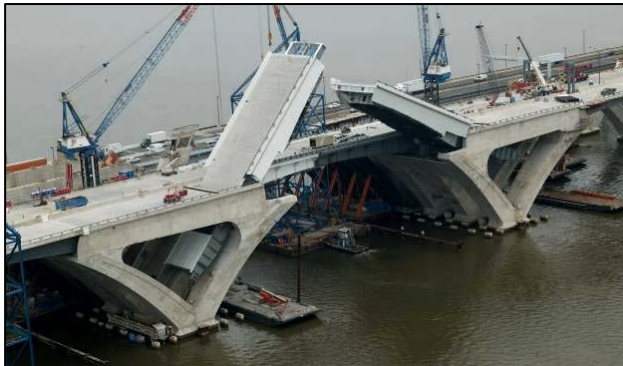
Fig. 5 Photo of bascule span construction
