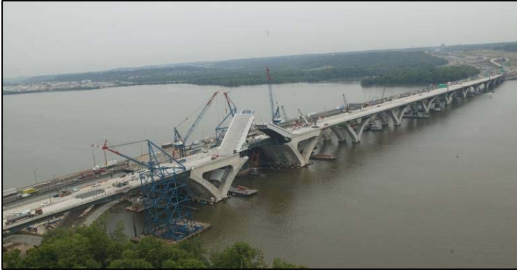
Fig. 1 Photo of the new bridge construction
