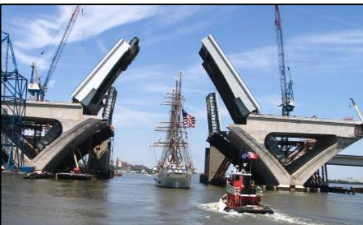
Fig. 11 Bascule span opening for ship passage
